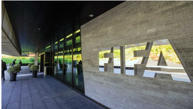
Figure 1. FIFA Headquarters, Zurich, Switzerland
